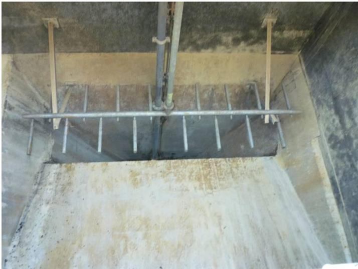
A second filtration step removes grit. Above is an image of the empty grit-removal machinery. The pictured bar rotates, which agitates the water and forces the grit to settle as the lighter water remains above.
