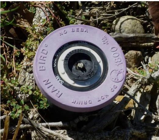
Purple coloration required for marking sprinkler heads using non-potable water.
