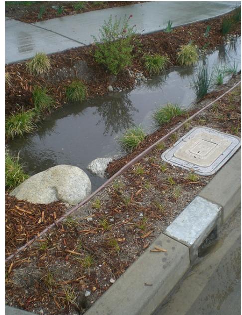
Figure 6.5: Bioswales capture and retain water for infiltration. Photo taken from Council for Watershed Health
