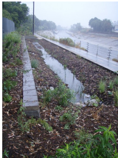
Figure 6.4: Rain Gardens, recently installed atop Ballona Creek, during a rainstorm. Photo courtesy of LACreekFreak.wordpress.com
