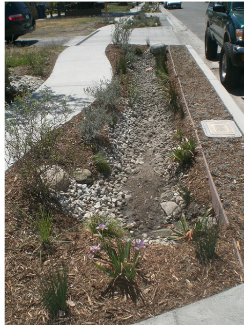
Figure 6.6: Elmer Avenue Bioswales aid in the infiltration of runoff while improving the aesthetic and walkability of the neighborhood. Photo taken from Council for Watershed Health
