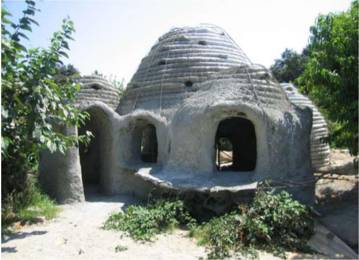
Figure 3: The second Earth Dome at the Pomona College Organic Farm in July 2005. Note the tubes of soil, the rebar and wire mesh, and the first layer of gunite on the bottom half of the structure. [http://en.wikipedia.org/wiki/File:Front\\_of\\_dome.jpg](http://en.wikipedia.org/wiki/File:Front_of_dome.jpg).
