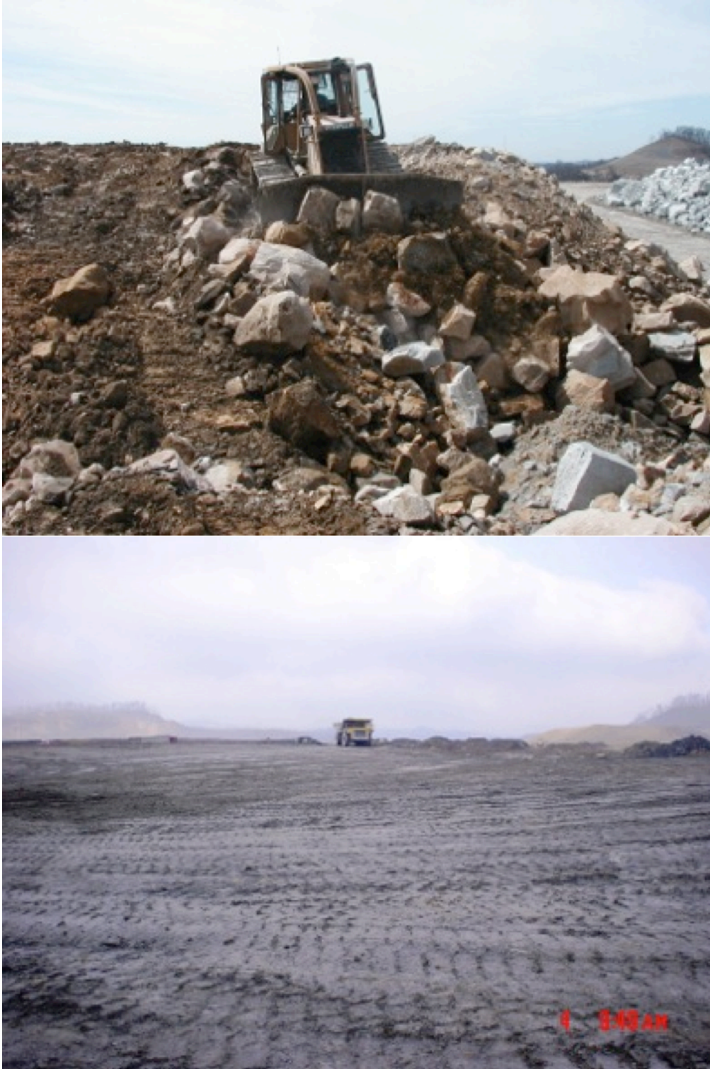
Figure 4. Surface mines partway through the reclamation process. By use of heavy machinery, the ground is highly compacted (above). While this temporarily improves land stability, it is not a conducive medium for plant growth, especially native tree growth (below).
