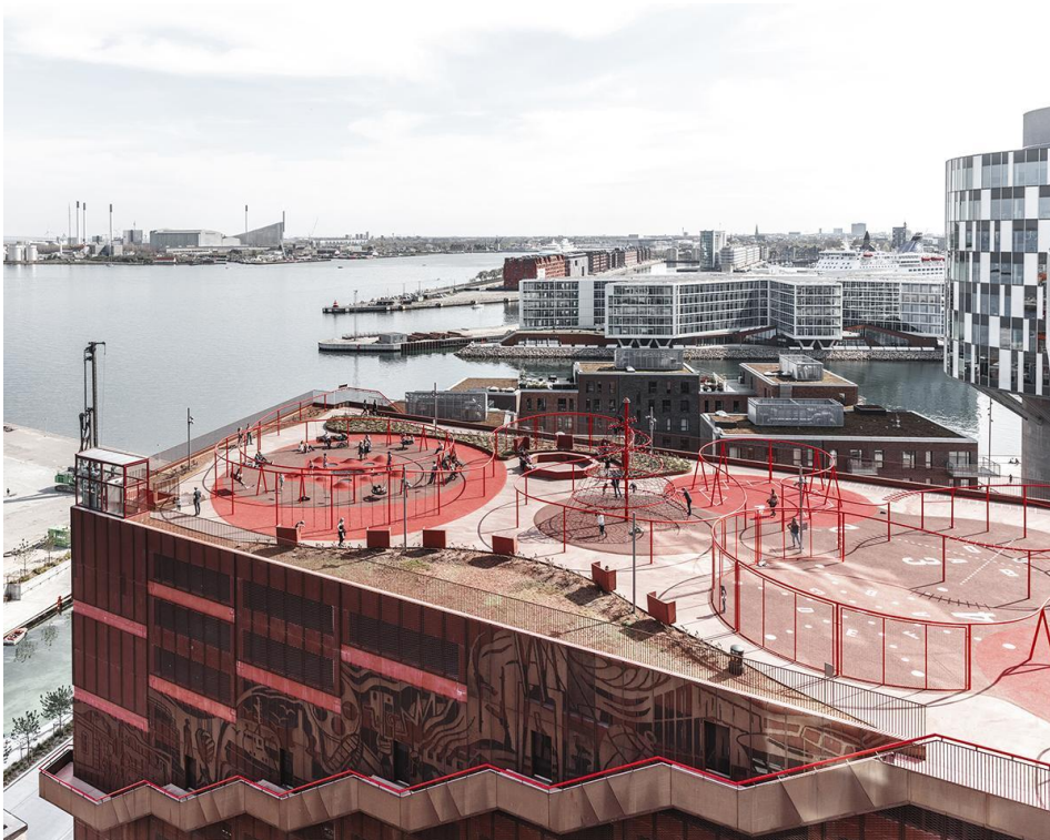
Rooftop view of Konditaget Lüders parking garage
