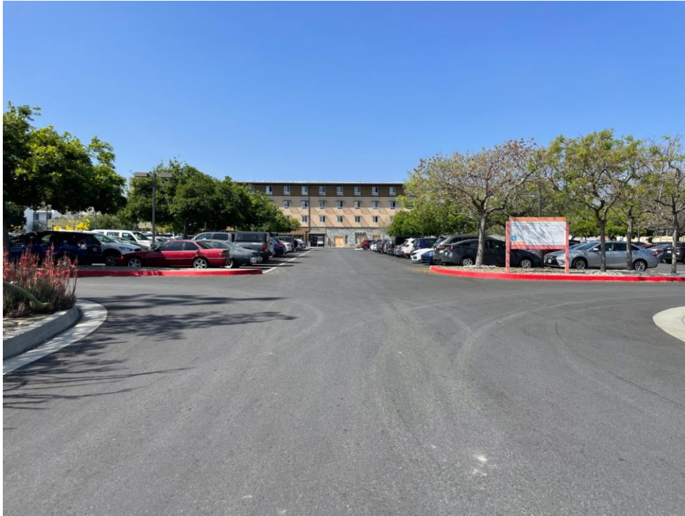
Current site entrance - Southern edge, bottom of grade
