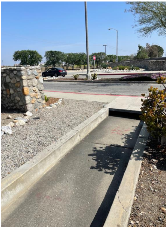
Drainage area - Southeastern corner of East Mesa parking lot
