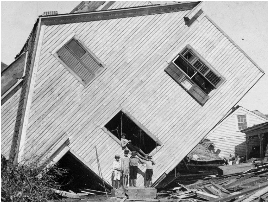
FIGURE 9. THIS IMAGE DEPICTS A GROUP OF CHILDREN POSING IN FRONT OF A HOUSE THAT WAS STRIPPED FROM ITS FOUNDATION AND SHIFTED BY THE HURRICANE'S WINDS. / LIBRARY OF CONGRESS
