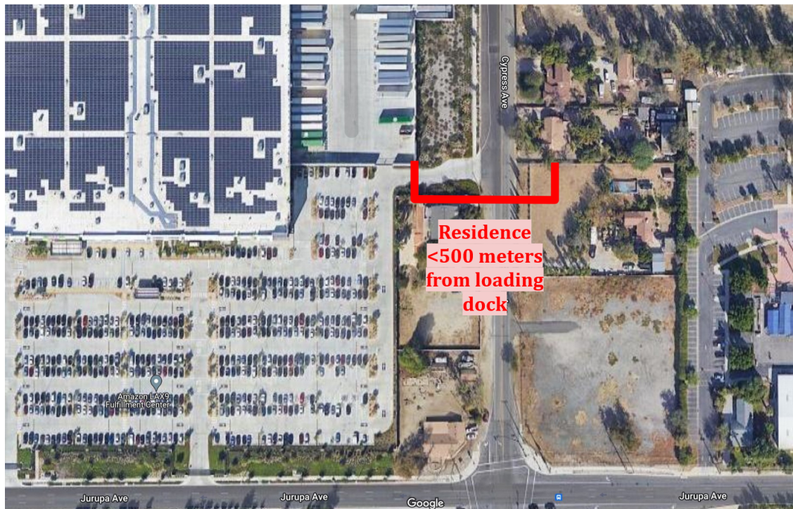
Figure 4.4: The southeast corner of Amazon's LAX9 fulfillment center. Residents who declined to sell their homes are now located only a few dozen meters from the loading docks, where an estimated 2,300 diesel truck visit every day (Wulfraat, 2022). Image courtesy of Google Earth Pro (Google, 2022a)
