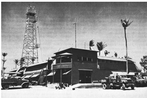
Figure 3. Quonset-Hut Variation at Eniwetok Base. Courtesy of Naval History and Heritage Command and the National Archives.
