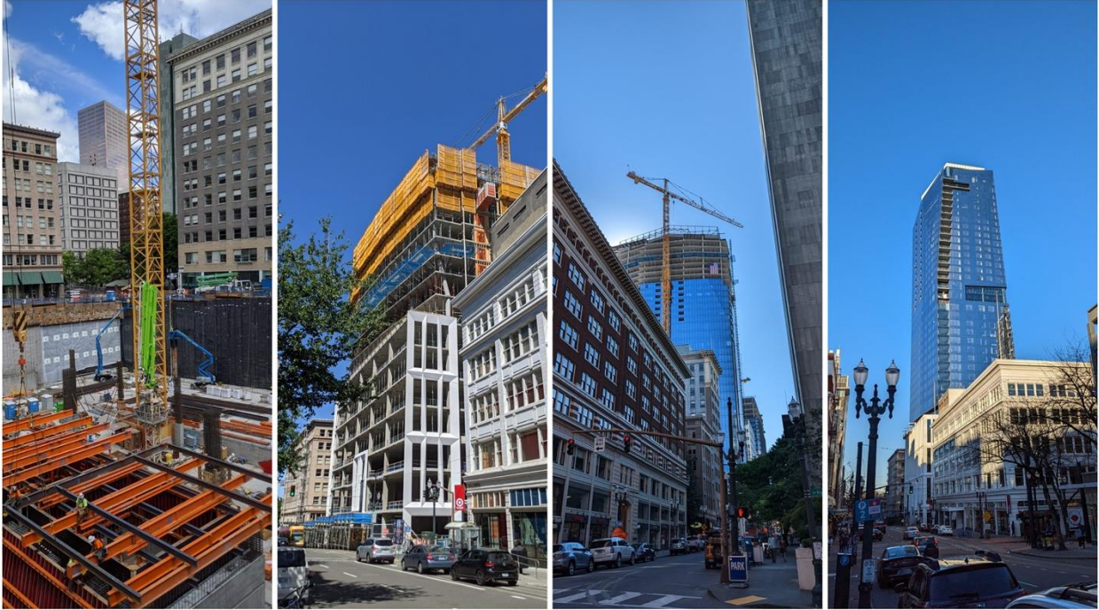
Figure 2: Block 216 construction photos (photos credit: Cello Expressions Photography)
