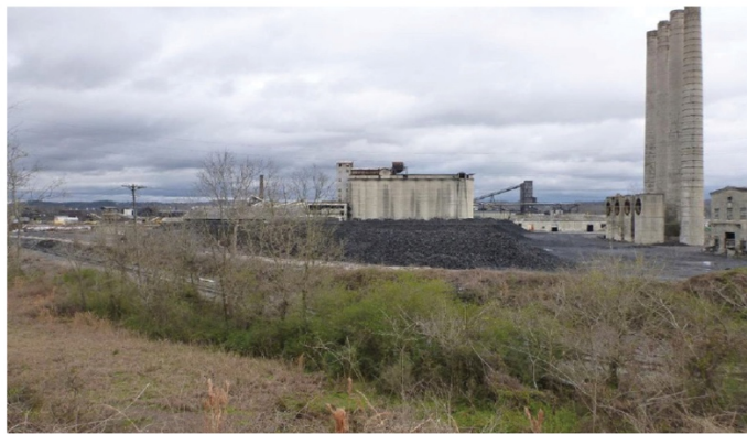
The now closed Wagner Laboratory located in south Springside was the site of missile defense systems and rocket engine testing and manufacturing between 1951 and 1994.
