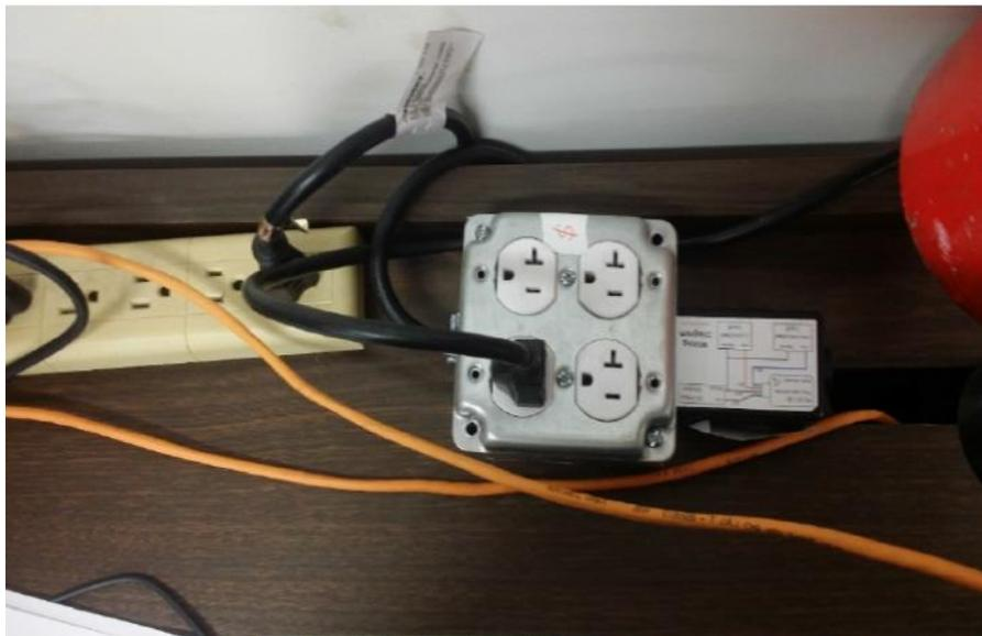
FIGURE 14: Enlighted Plug Load Controller installed at ECS 411.
