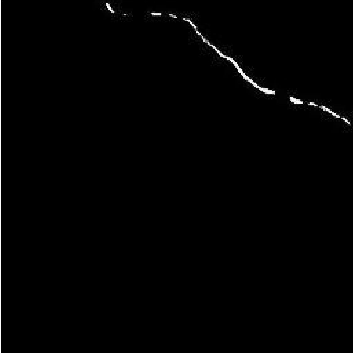
Figure 7.13: Merged Upper and Lower Edges of Wall Crack After Applying Optical Flow Warping
