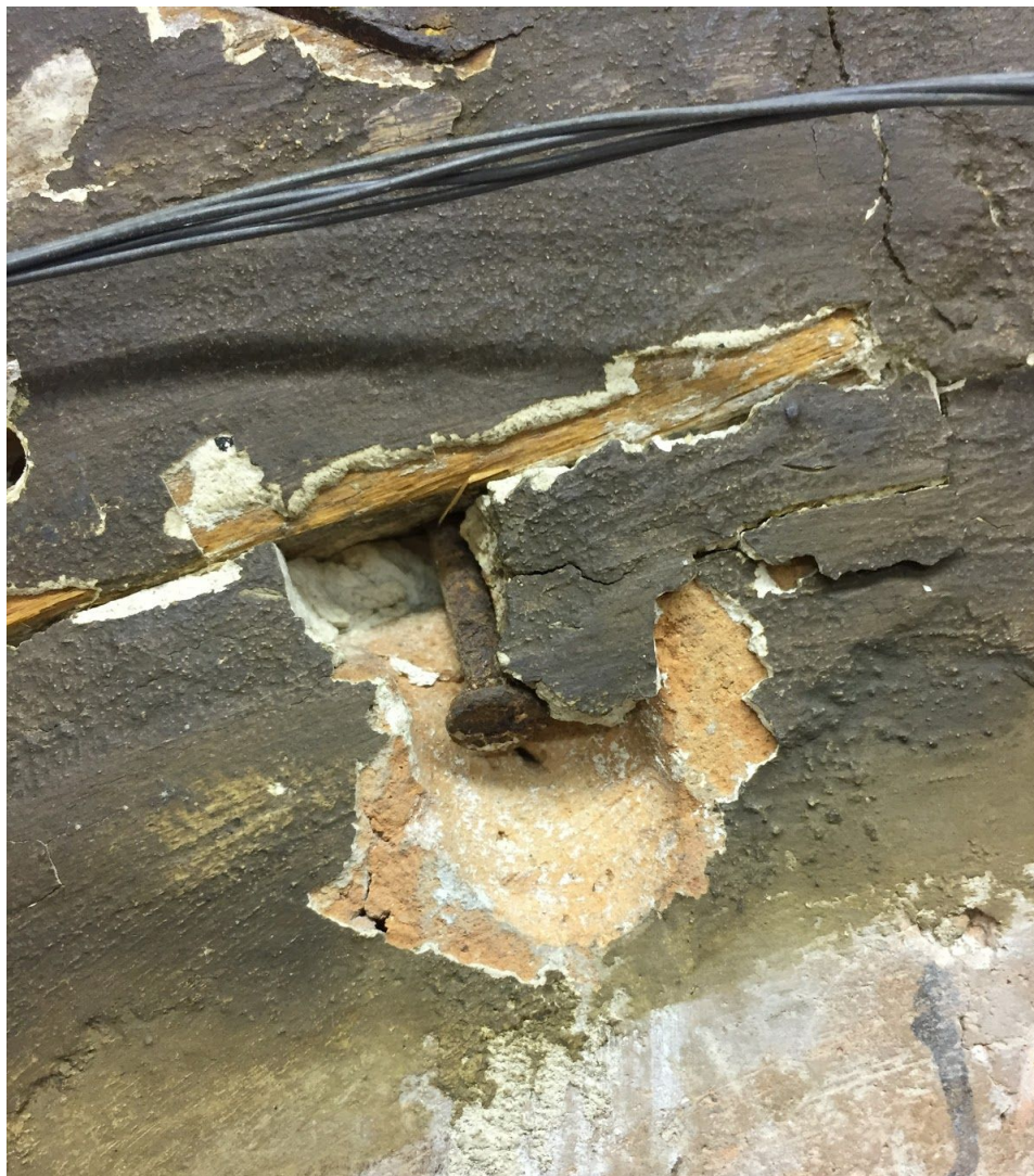
Figure 3: Calligraphic Roundel, Detail of nail between the frame and ceramic roundel, Reverse. Exhibited plaster layer cracking and flaking. Source: Josephine Ren.
