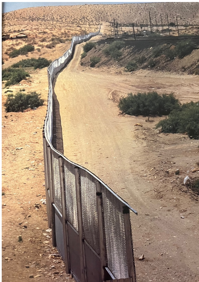
Constructed in 1997 as part of Operation Hold the Line in New Mexico. In Bowden, Charles. "Juarez the Laboratory of Our Future," 37.
